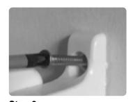
**Step 3**Use screw driver to fix the screws into the wall.
